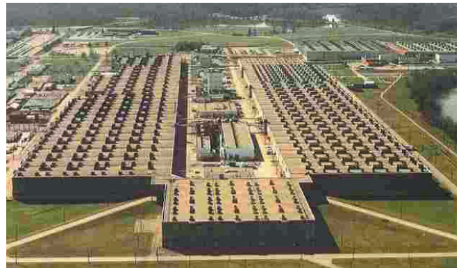
The Original K-25 Gaseous Diffusion Plant.
