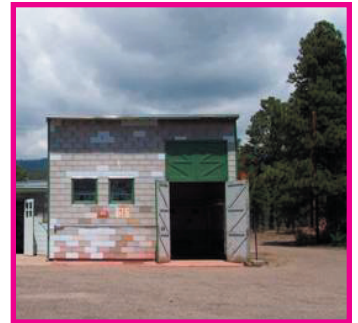
V Site After Restoration. Photo courtesy of LANL.
