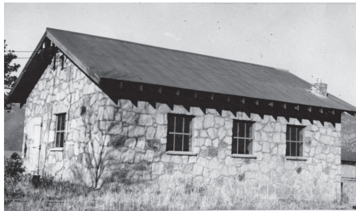
The Stone Power House at Los Alamos
